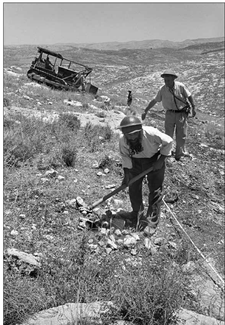
Workers build the “Burma Road” between Jerusalem and Tel Aviv, June 1948. (© Robert Capa, © International Center of Photography/Magnum Photos.)
